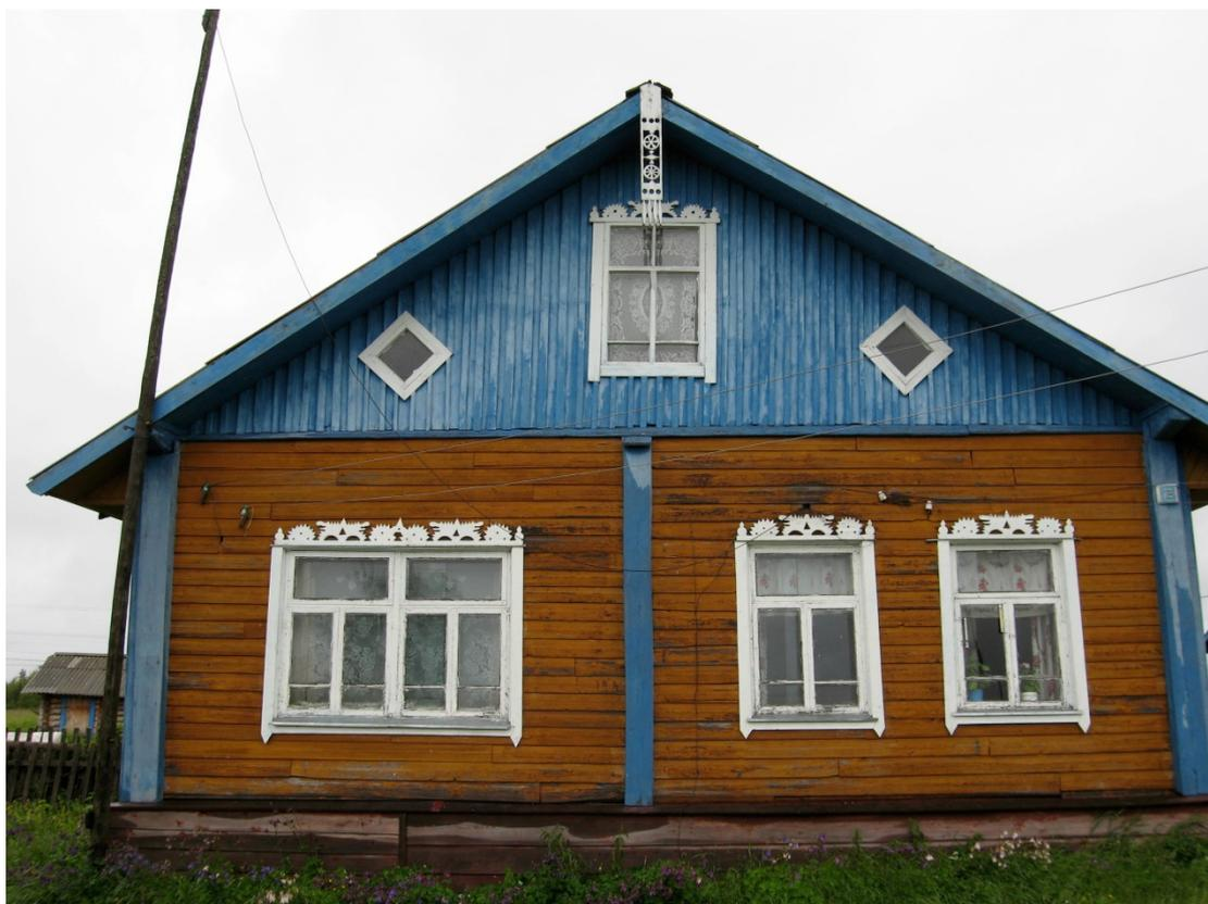
Figure 8: A nineteenth-century house in Jyskyjärvi village, Russian Karelia. It illustrates how a light timber structure, lacking ground-set foundations, can be well-finished and decorative, with architectural pretensions. Like the hall-type buildings on post-Roman sites in northern and western Britain, its archaeological traces would be fugitive. (Photograph John Blair.)
